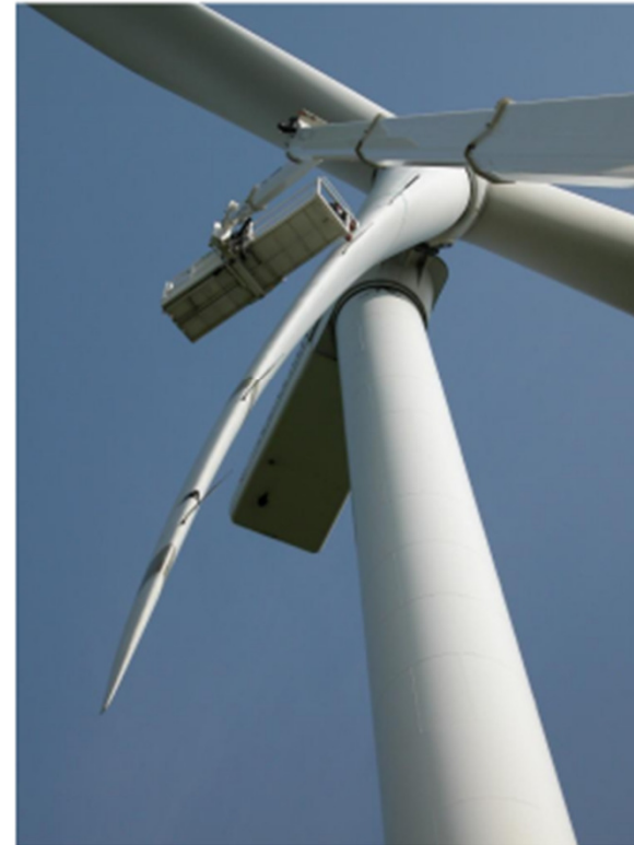
4 pitot tubes on the 80m, 2MW, NM80 turbine
